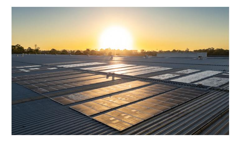
Modern BIPV systems are, to put it simply, solar building materials; they are roofs, tiles, windows or facades that serve as an outer layer for the structure while generating electricity for on-site use or export to the grid.
